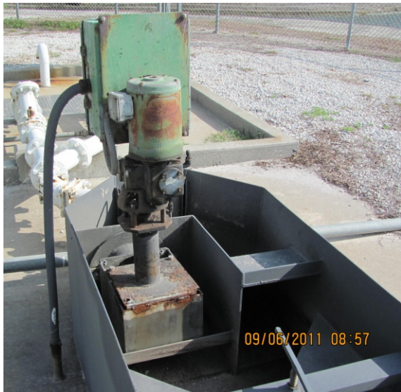
REPLACING ORIGINAL CLOW A-8
